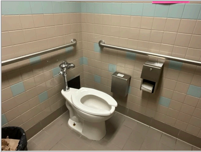
TOILET STALL OVERVIEW
