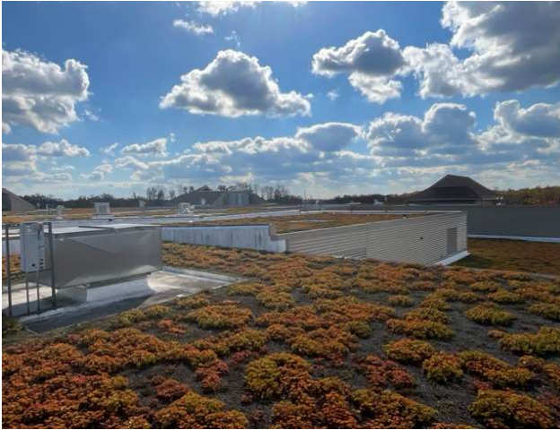
7 - PRIMARY ROOF OVERVIEW
