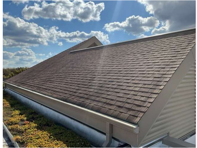
8 - SECONDARY ROOF OVERVIEW
